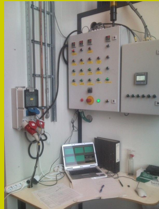
Engine control & monitoring
